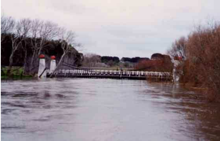
A flooded Merri River – Wollaston Bridge August 2001
