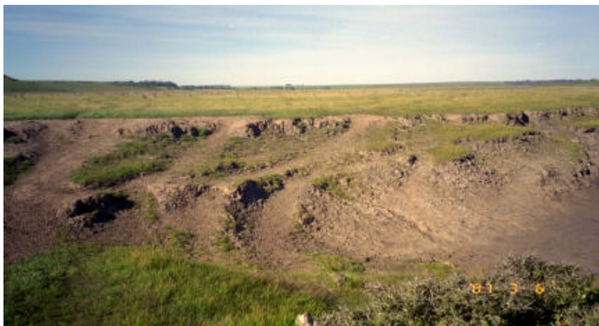
Figure 11: Basalt Plains - on-ground works in the region are targeting areas to increase bank stability (2000).
