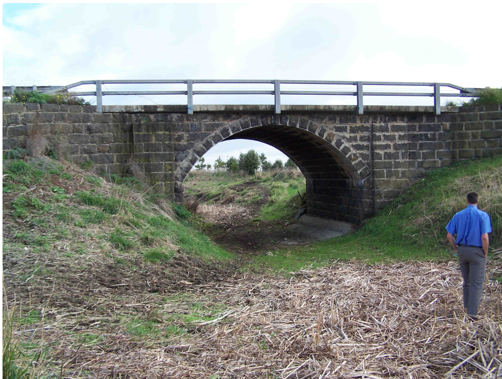
Figure 2-4 Bluestone Arch under Penshurst-Port Fairy Road at Murray Brook
