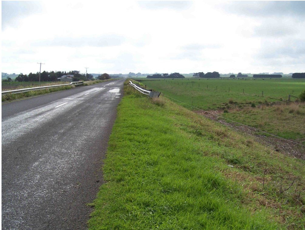
Figure 2-3 High Embankment, Resulting in Constriction Through Floodplain (Penshurst-Port Fairy Road at Murray Brook)
