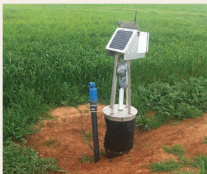
Automated pipe and riser irrigation system. Photo: GBCMA
