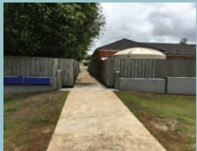
Figure 13: Blue boards on left of access can be inserted to fill the gap in the flood wall (photo by Johanna Theilemann)
