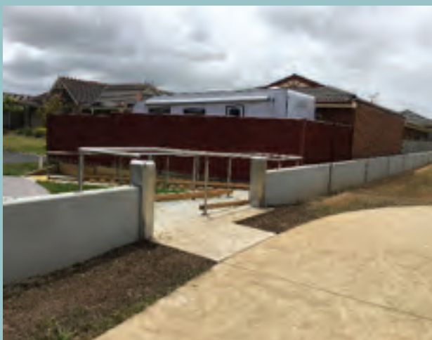
Figure 12: Flood Wall with pedestrian access at Russell Creek (photo by Johanna Theilemann)
