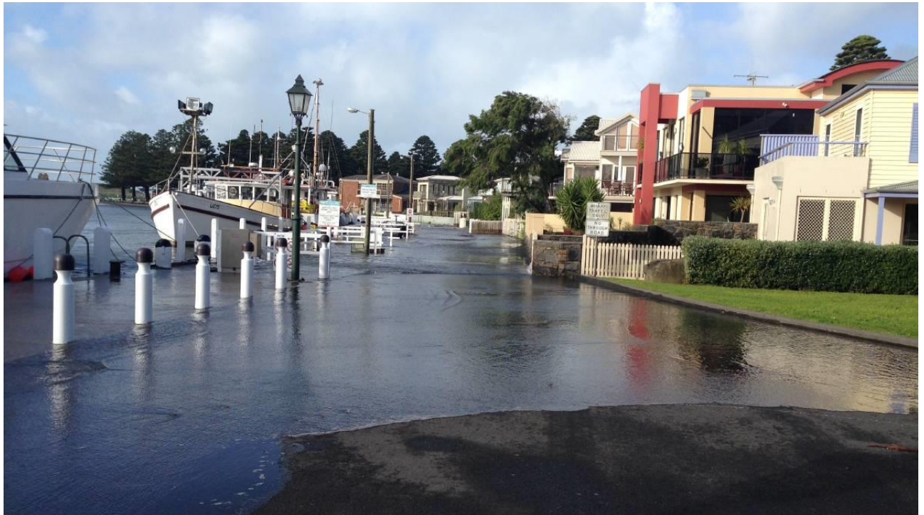
Figure 17 Water over the accessway beside the Port Fairy wharf during the June 2014 flood event (Courtesy of the Warrnambool Standard)
