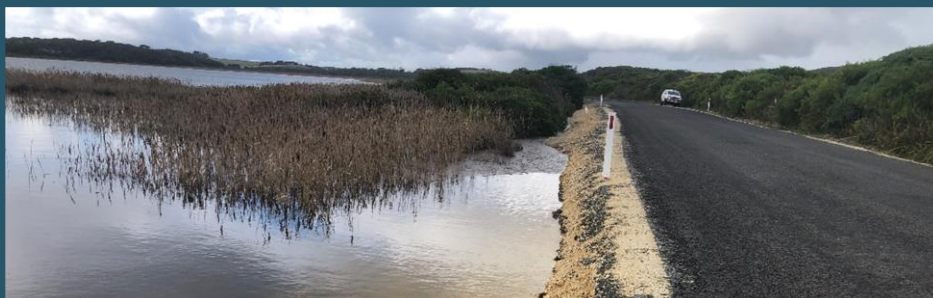
Beach Road, Nelson (Glenelg Estuary) was raised in elevation in 2024 to maintain visitor access during increasingly frequent estuary inundation due to estuary mouth closure. Credit: G Prentice.
